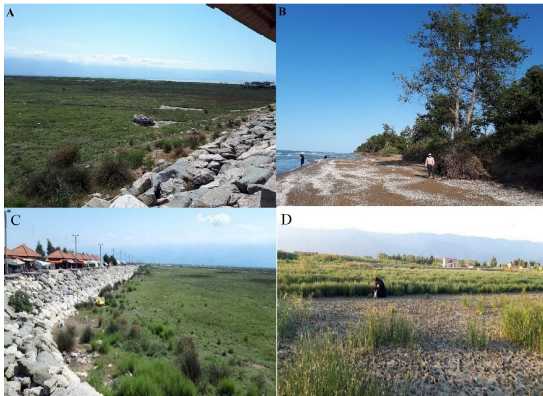
Fig. 6. A: shoreline Progression in Bandar-e-Turkmen, B: erosion of coastal area due to port construction and decrease longshore drift in Miankaleh, C: water regression beside Bandar Turkmen break wave and D: Bandar Gaz port floor covered by vegetation due to water regression (All picture captured in 2020)
