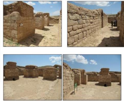
Fig. 4. The stone blocks used in the northern hall of the Khosrow portico
